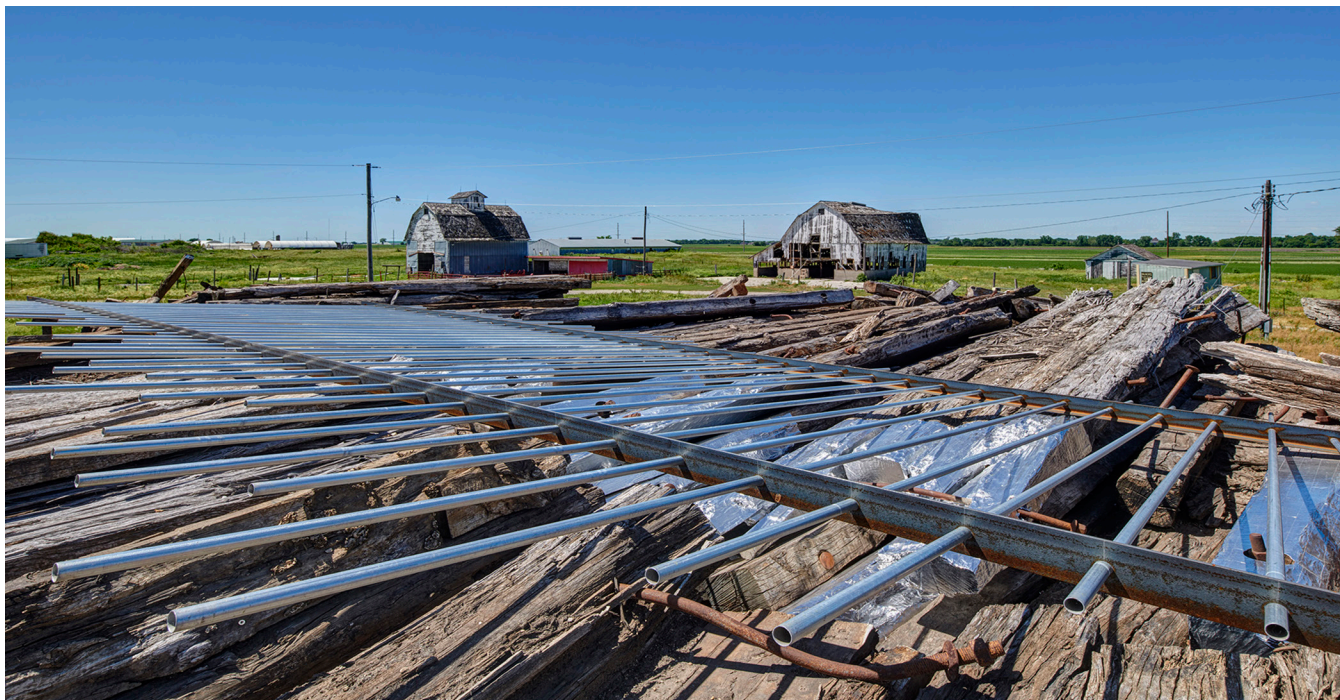
Figure 9. View atop looking north. Photography by Integrated Studio.
